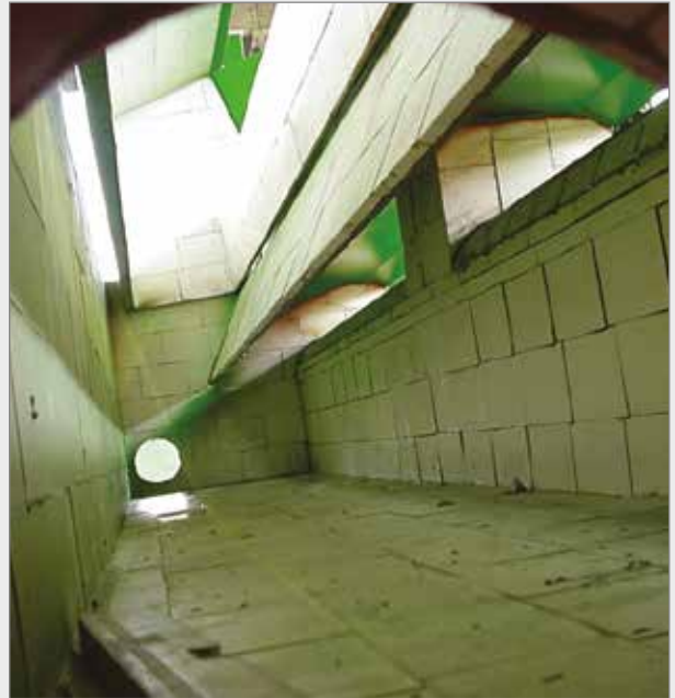
Stilling feed chute lined with ceramic tiles (optional rubber lining).
